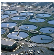
Stormwater & Wastewater Treatment Facilities
