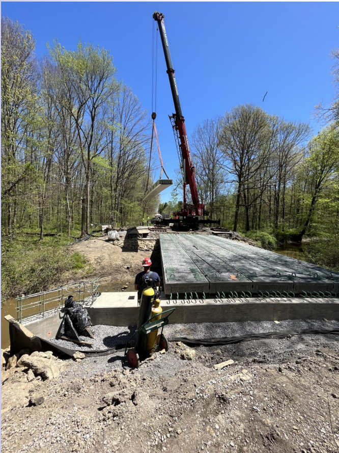
FAR #16 BRIDGE REPLACEMENT HOUSEL CRAFT RD.
